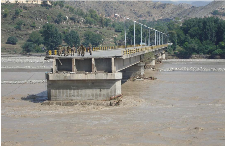
Chakdara Bridge - Malakand
